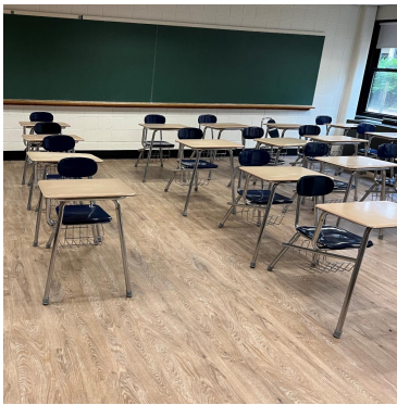
Repairs included new flooring in some classrooms.
